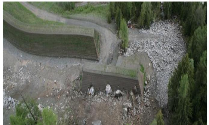
and rockfall events without the need for repair. Given enough space, almost unlimited energy absorption capacities are achievable. An example of such concrete reinforcement that can be deployed in Swat is shown in picture.
